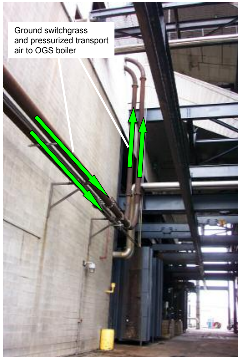
Switchgrass Blow Lines Transporting Ground Switchgrass into Boiler House (left) and Boiler (right).
