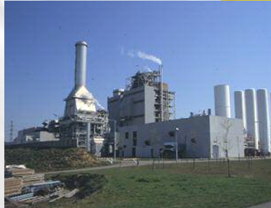
250 MW e Integrated Coal Gasification Combined Cycle plant, Willem Alexander Centrale
