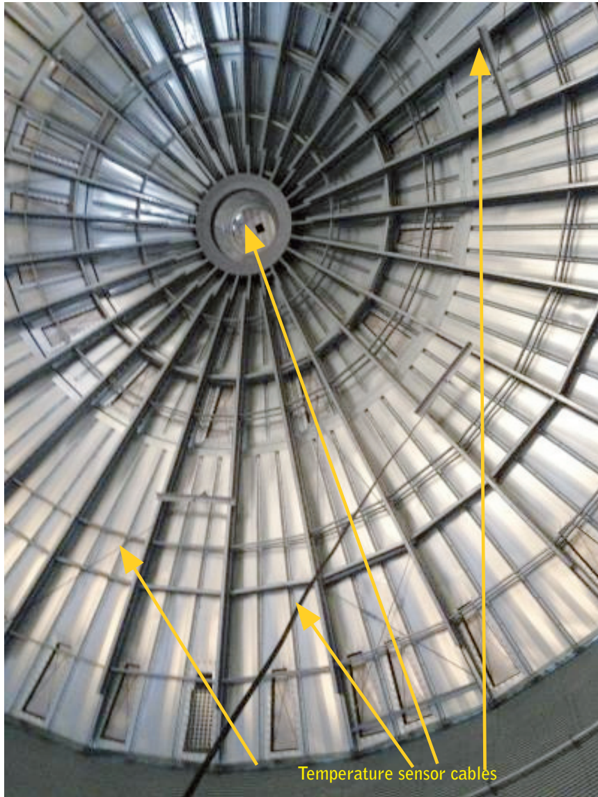
Figure 3.16. Monitoring of the temperature trends inside bulk storage is important to indicate if there is an unusual self-heating on-going. The black lines from the roof in the picture show temperature sensor cables normally used for such monitoring. . This silo (20 m in diameter) is equipped with one line in the silo centre and six lines distributed at half the radius. All together the seven lines include 37 temperature sensors which are connected to a control system. (Photo Anders Lönnermark, SP)
