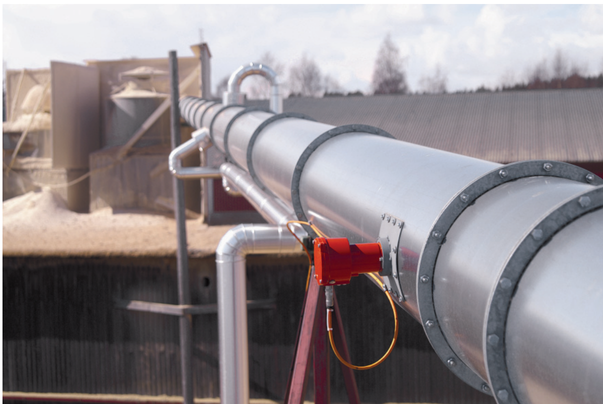
Figure 3.8. A detector indicating sparks and hot particles in a ventilation duct. These detectors are often connected to a fast activating water spray system downstream the detector (not in this picture) (courtesy of Firefly).
