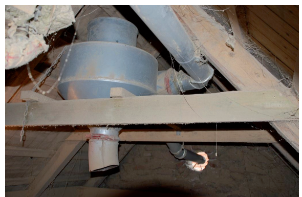
Figure 8.7. A better way to deliver pellets to a private end user compared to Figure 8.6. The pellets are blown from the truck in the pipe at the top of the picture and delivered to the silo through the open pipe in the bottom of the cyclone. The transport air is separated from the pellets in the cyclone and is blown in a tube through the hole in the wall to the open air far away from the truck and the driver [158].
