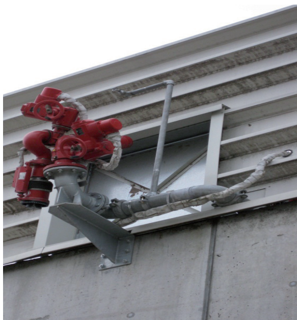
Figure 3.13. Example of a remote controlled water cannon installed on the capstone of a fuel storage facility for a first fire extinguishing [86].
