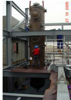
Gas cleaning equipment inserted – 27th October 2005
