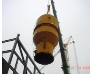
Gasifier unit produced in Finland while inside brickwork is performed by Finish and Danish Companies
