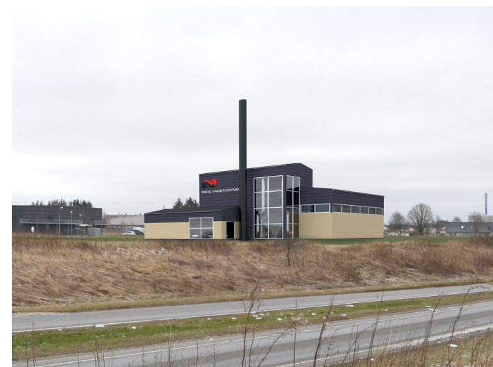
The CHP plant in Sindal at inauguration in September 2018.
