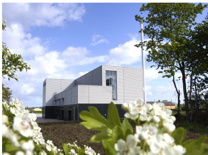
Dall Energy plant in Sønderborg (9 MW heat-only).
