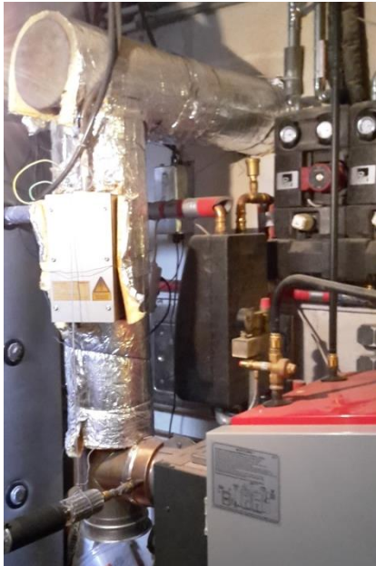
Atmos, wood chips 18 kW
